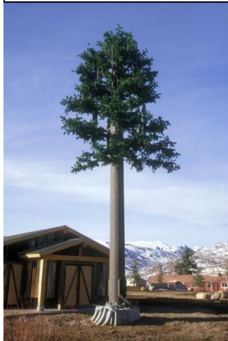
Photograph shows an example of Stealth Technology. Source: http://www.telepp.com/support/photos/monopine.jpg
