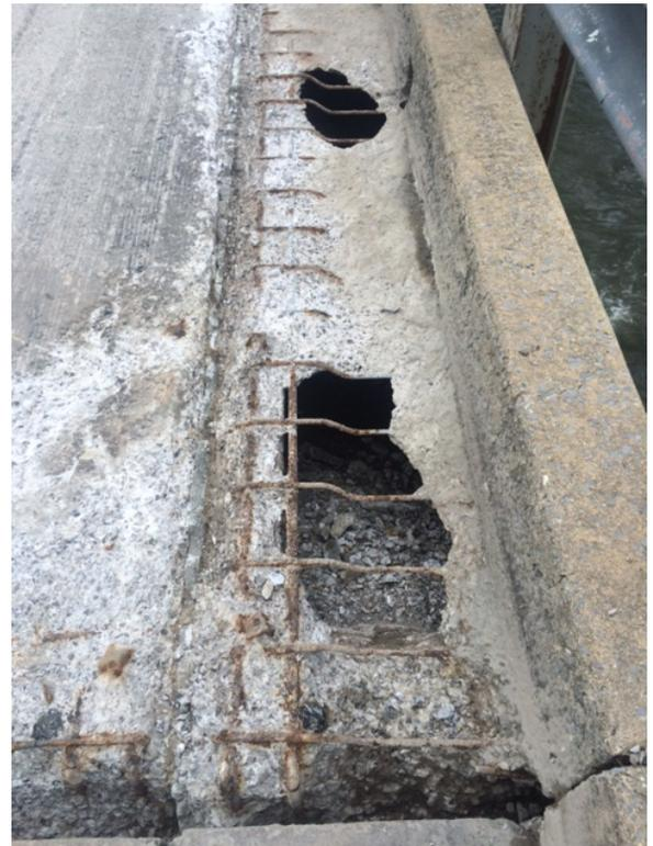
**Beam deterioration on Bergner Bridge. The holes in the beams will be repaired as part of the additional maintenance work.**
