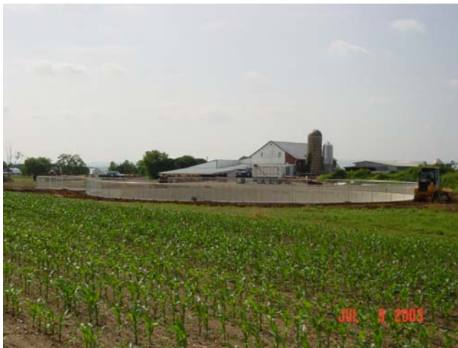
Newly Installed Waste Storage Structure
