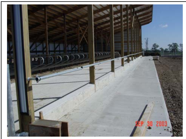
Concrete flooring was poured at heavy use areas
