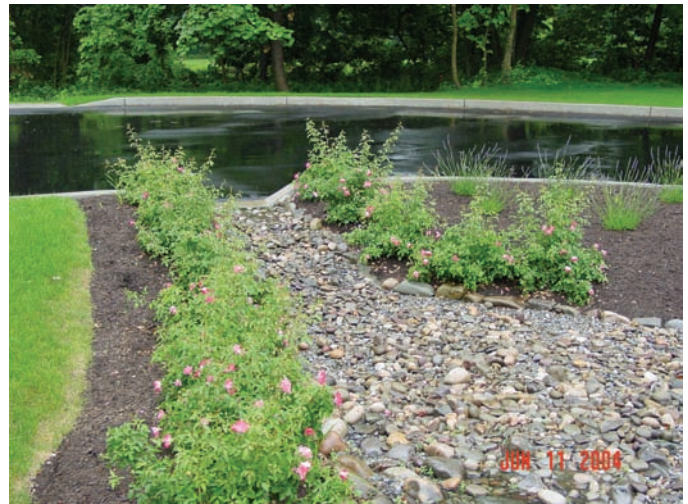
Bioretention/infiltration area receiving runoff from a paved drive.
