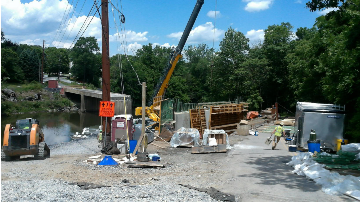
Abutment 2 Construction - Looking North -
