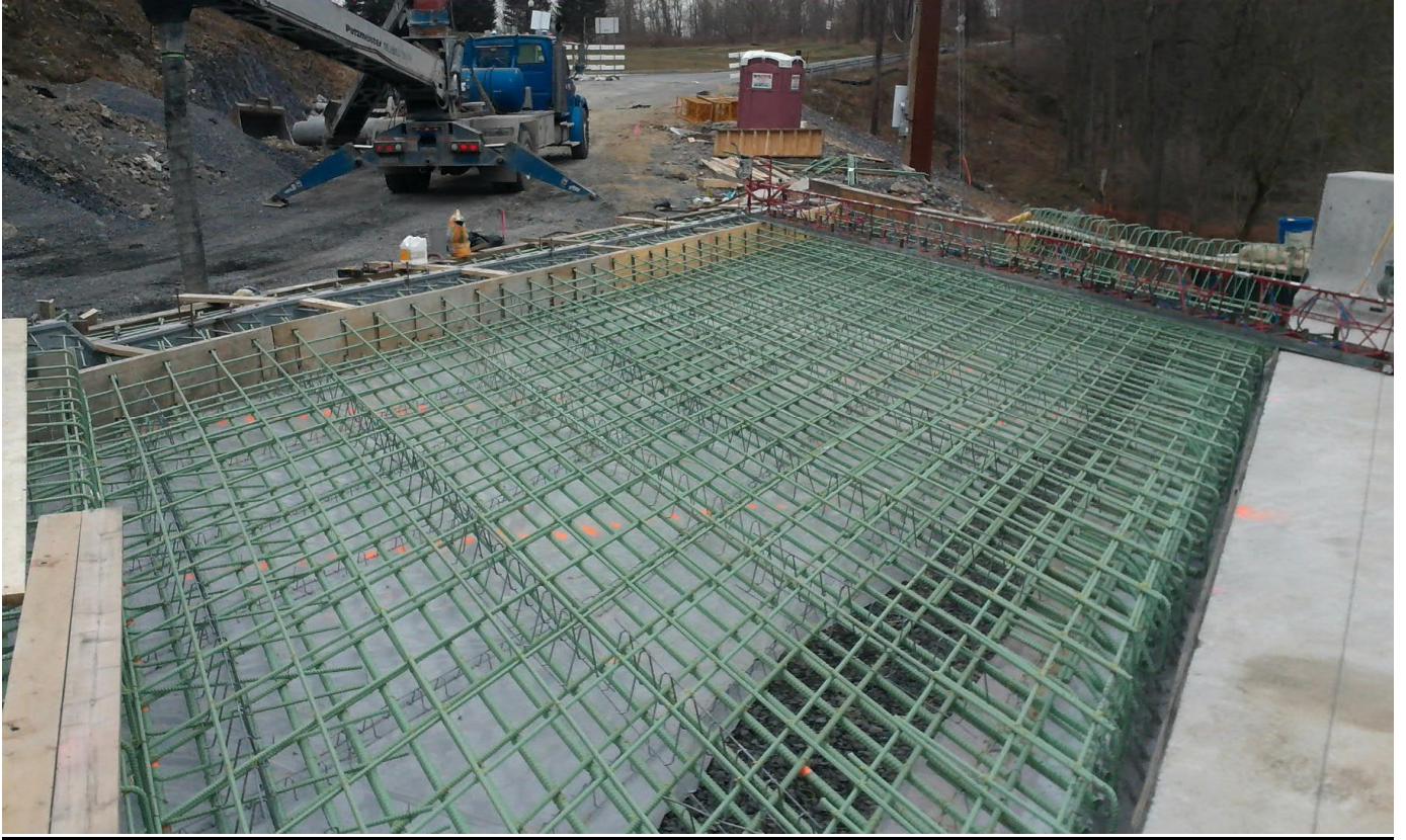
Approach Slab Rebar Placement (Looking North)
